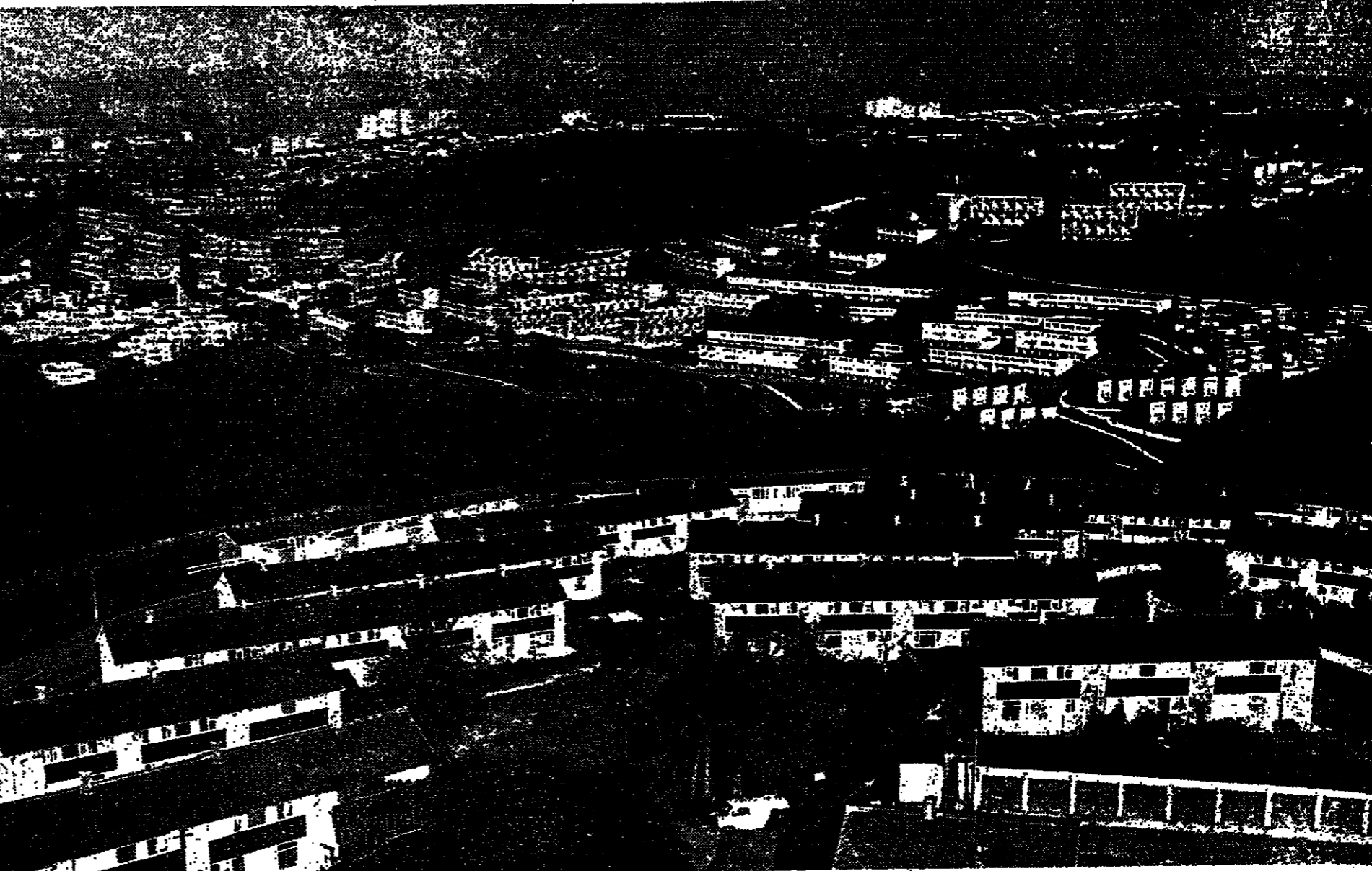
The Gleadless Valley housing development is built on a steeply sloping hillside only one and a half miles from Sheffield city centre.
